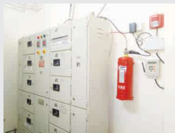
FIREDTK Tubing Installation
